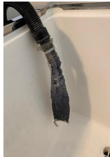
Left Photo is a newly installed Lint Catcher.....Right Photo is a Lint Catcher in need of replacement
