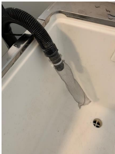
Left Photo is a newly installed Lint Catcher.....Right Photo is a Lint Catcher in need of replacement
