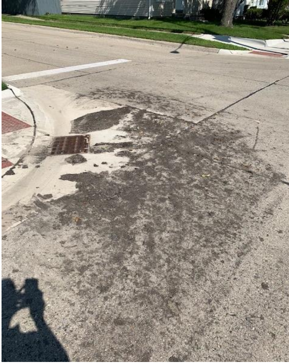
Post Storm - Landscaping Dirt
